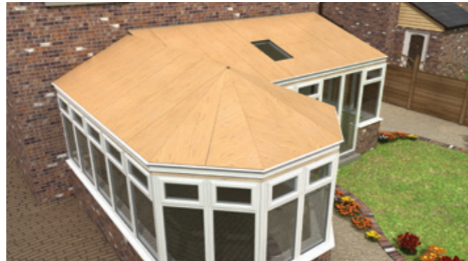
Exterior grade plywood is fixed to the rafters.
